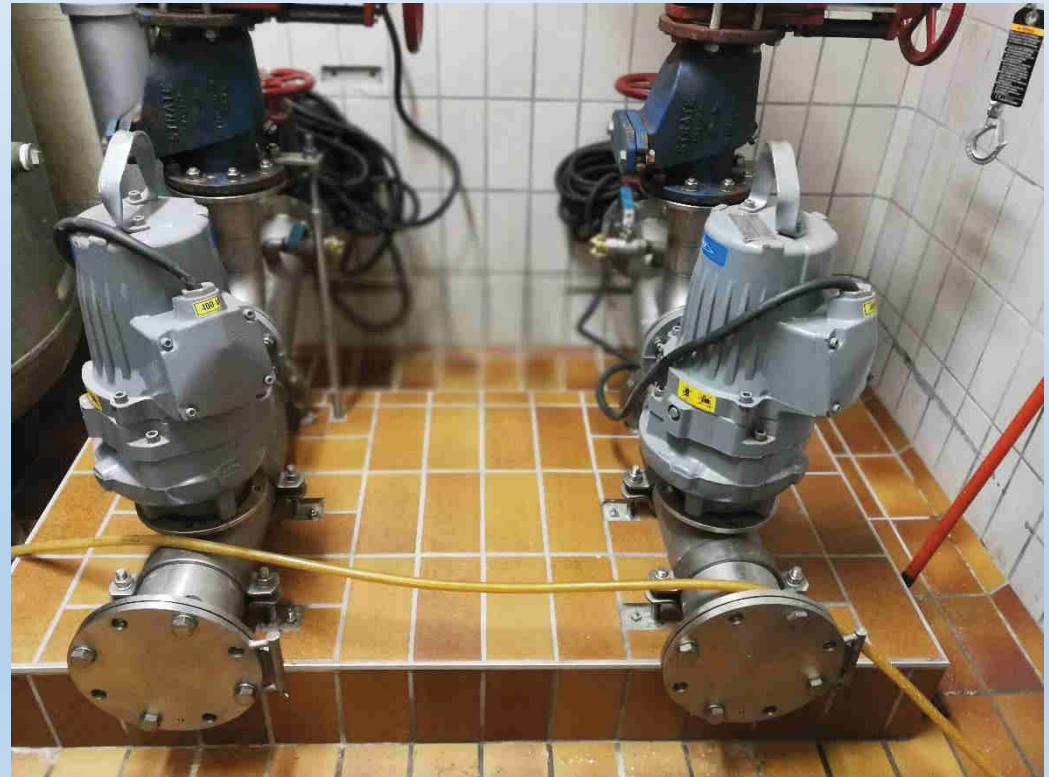
Pumpwerk Peterswörth Gries
